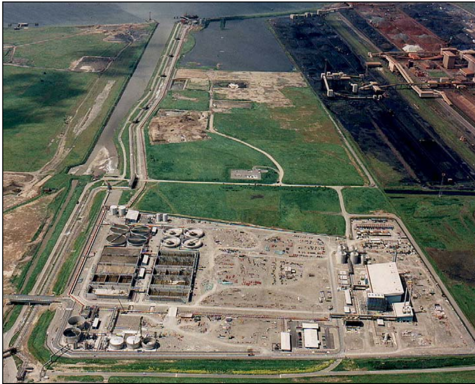
Figure 2: Bran Sands Development under Construction
